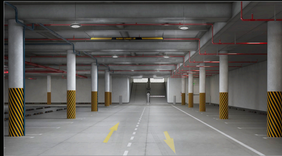
Two Lane Parking Garage
